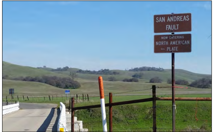
Earthquake capital of the U.S. Bridge on Parkfield-Coalinga Road straddles the San Andreas Fault. Photo taken by Carl C.de Baca
